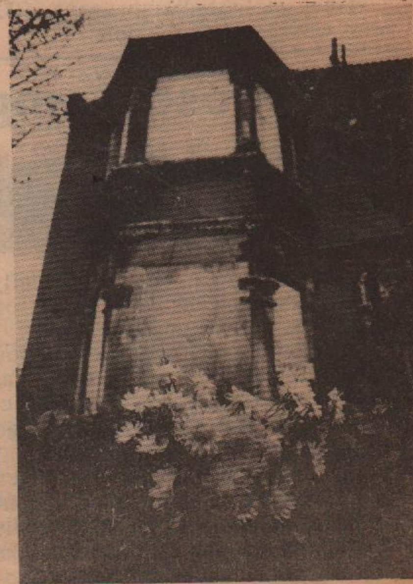
The house in Burgess Road photo: Jezz Coulson IFL
